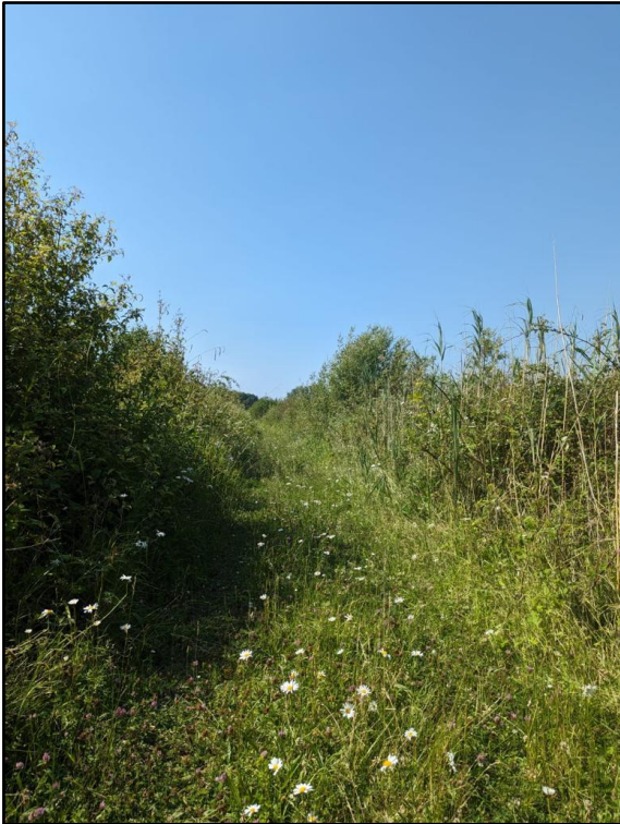
Plate 1: view of the bund looking north-west.
